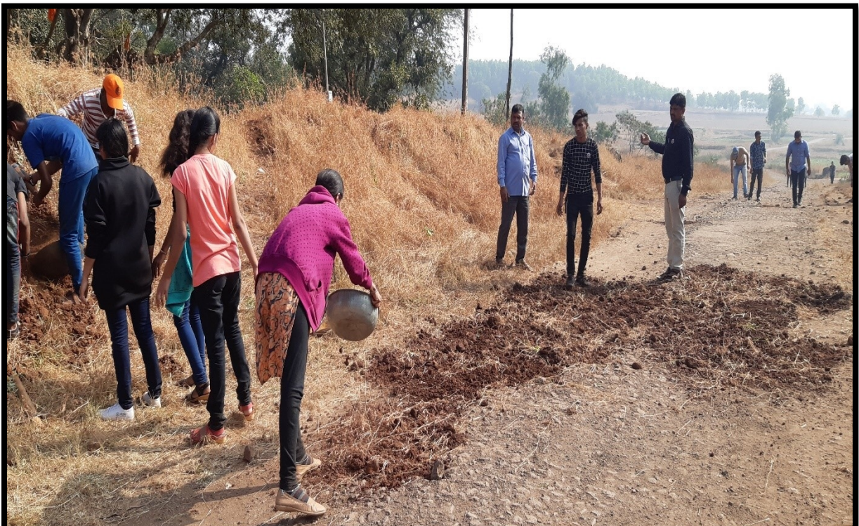
Road repairing in village
